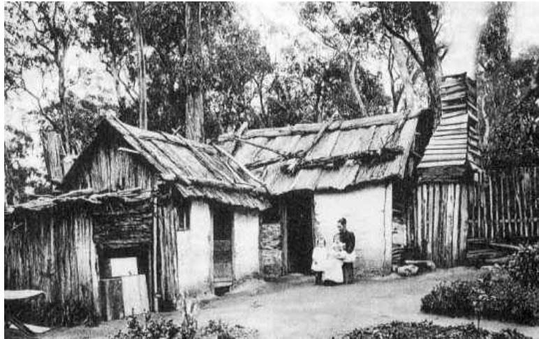
Wattle and Daub home with a bark roof and parget wooden chimney.
